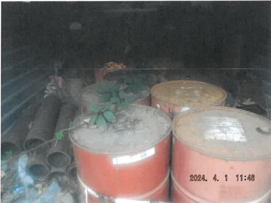
DSCF2899 - View of storage of waste hydraulic oil without adequate secondary containment. These drums were observed in a storage unit on site.
