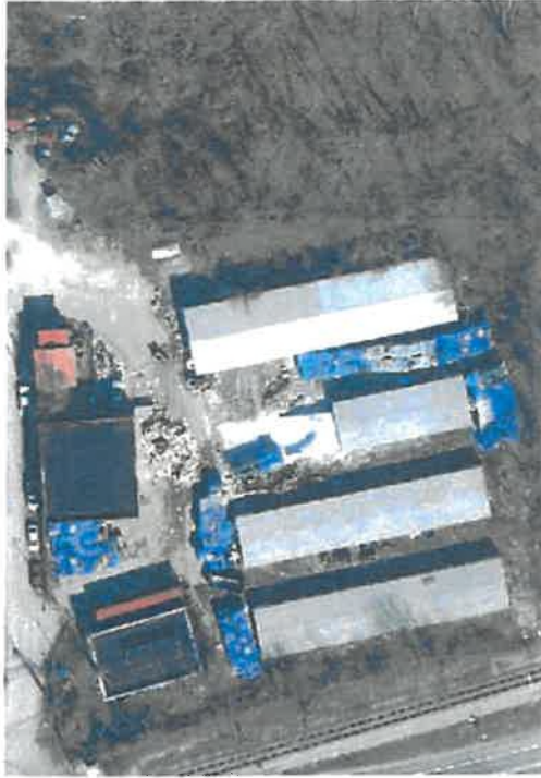
Overview of the recycling facility (image taken from WV Flood Map Tool).
