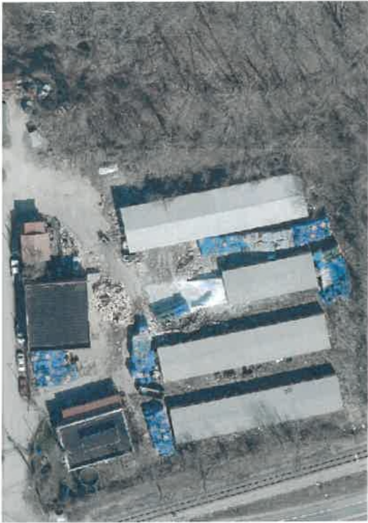
Overview image of the M&M Fibers recycling facility (image taken from WV Flood Map Tool).
