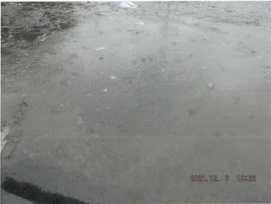
12.6.2021 – View of stormwater with a visible oily sheen and paper fibers draining into a drop inlet which is connected to an unpermitted point source (previously Outlet 001).
