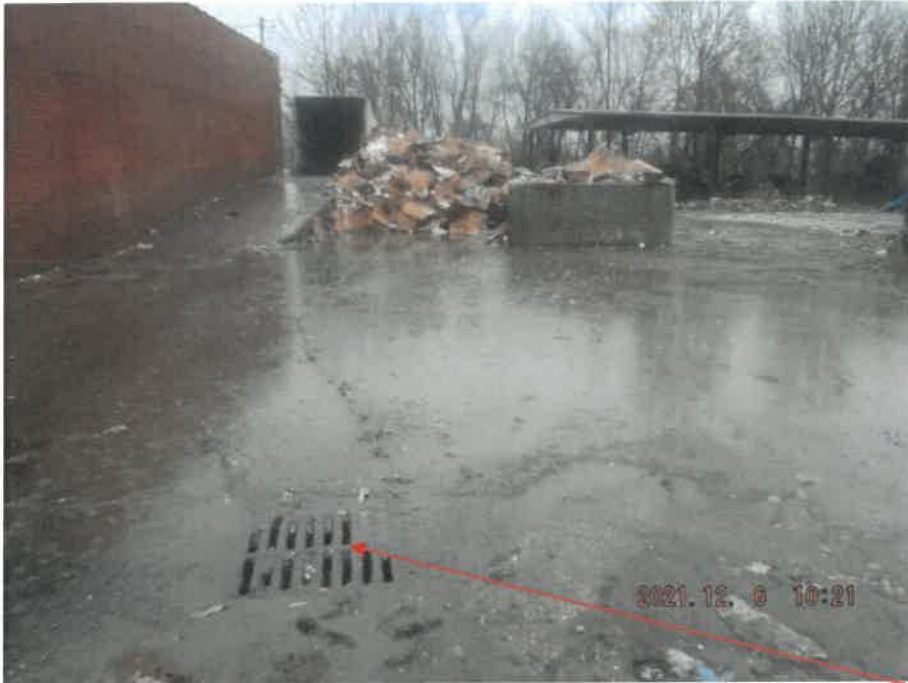
12.6.2021 – View of the property operated by M&M Fiber Recycle with a drop inlet that discharges to an unpermitted point source (previously Outlet 001).
