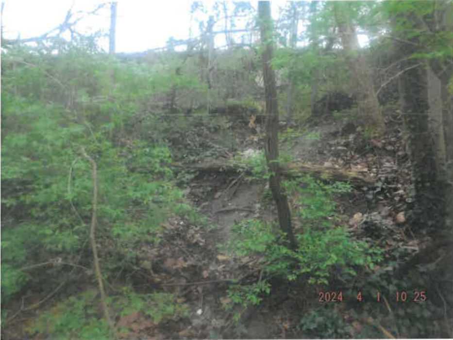
DSCF2891 - Overview of the unpermitted outlet area (previously outlet 001).
